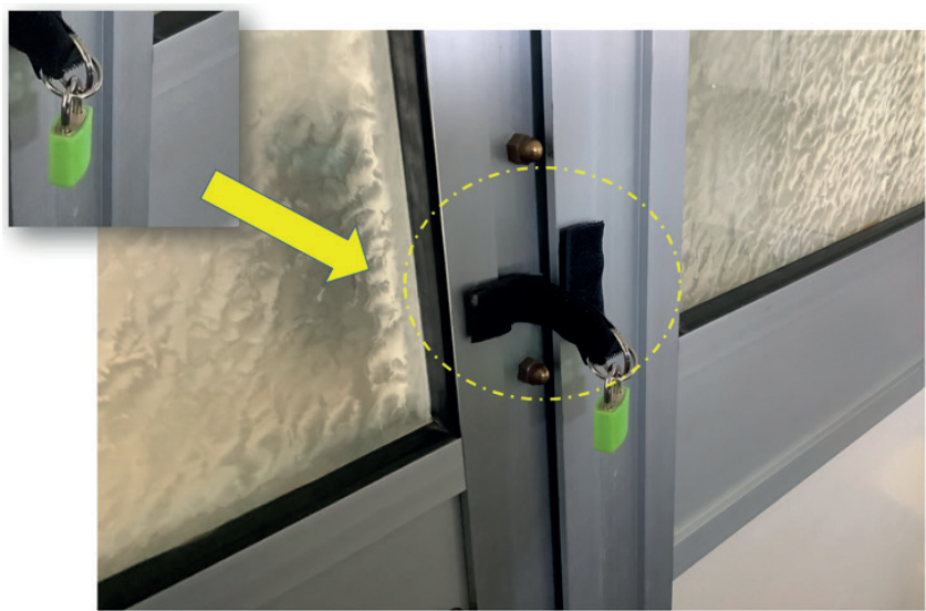
Photograph 4. Closure with ring devices fixed with velcro
