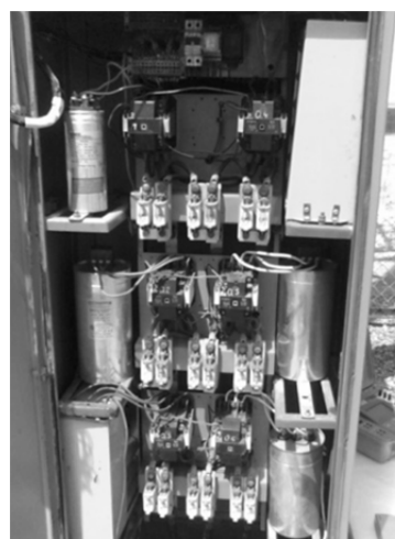
Fig. 1 A view of the compensation system with the energy capacitors (own photo)
