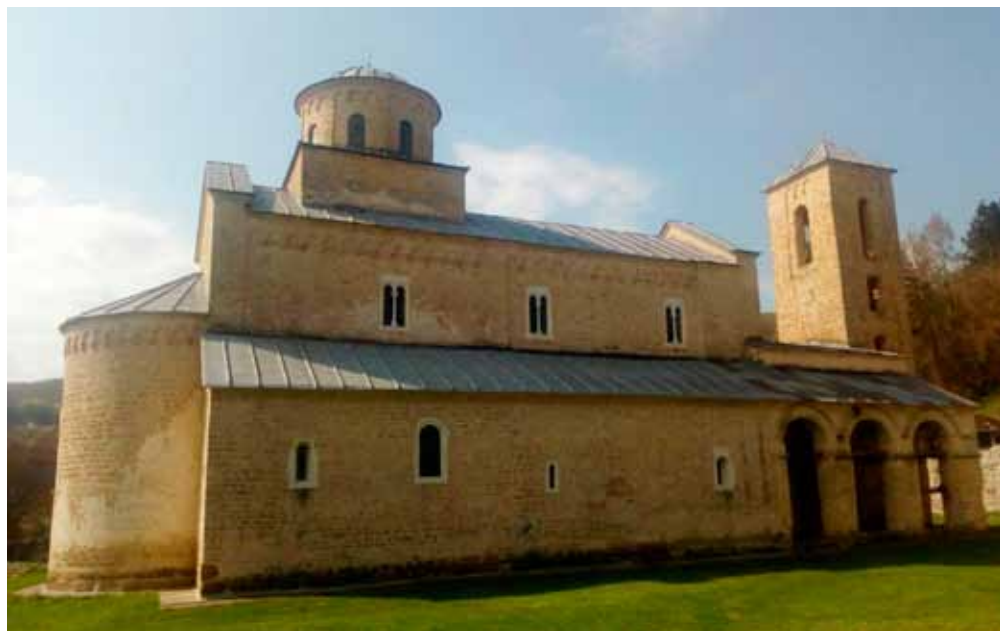
Fig. 6. Church of the Holy Trinity, 13 th century, Sopoćani monastery, view from the north (Photo by O. Špehar)
