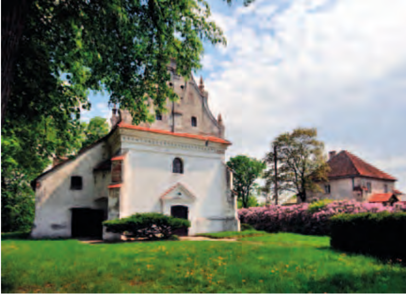
Fig. 6. View of St Anne's church from the north-east; the Tęczyński's manor is in the background (photo by P. Pytlak)
